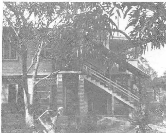
The lower part of the church building at Vreed-En-Hoop is being enclosed for additional space.
